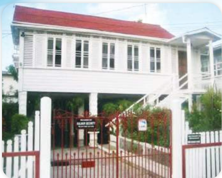
FIGURE 10: WOODEN COTTAGE ON MOULDED CONCRETE BLOCKS, MID 20TH CENTURY, GEORGETOWN
