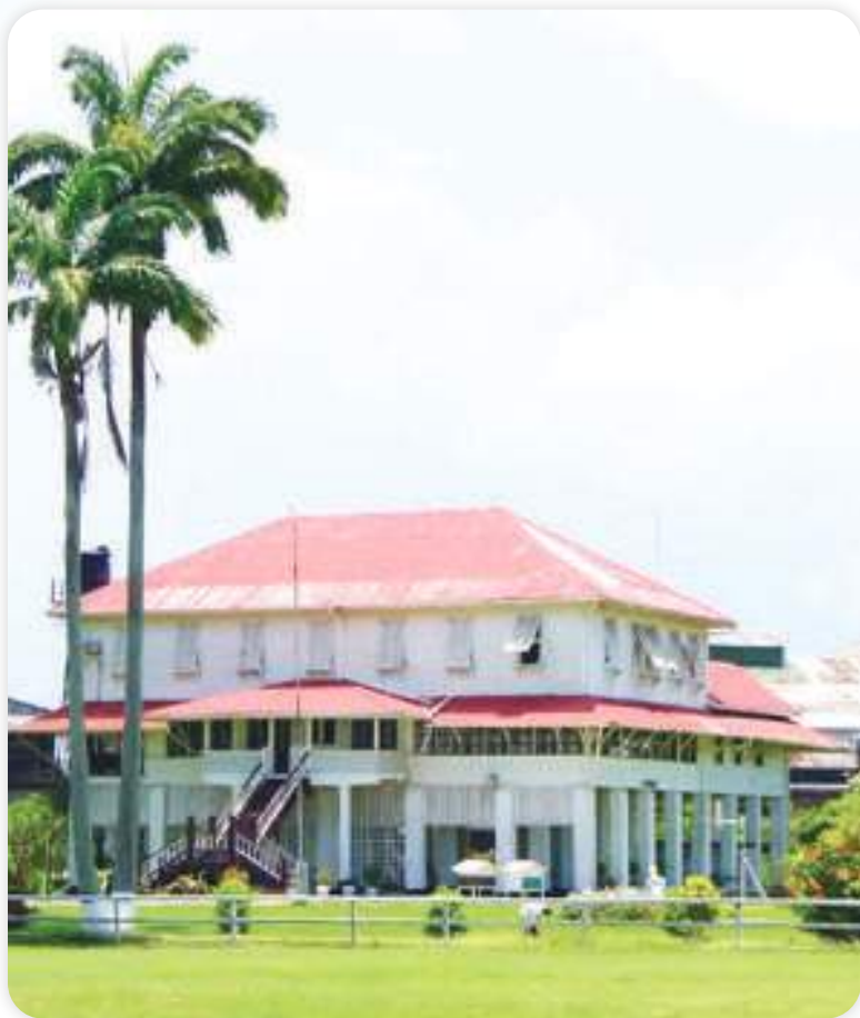
FIGURE 5: TYPICAL RURAL PLANTATION (ESTATE) GREAT HOUSE IN BERBICE, WITH HIPPED ROOF AND ON BRICK PILLARS, BUILT EARLY 20TH CENTURY
