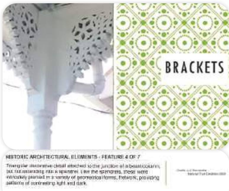
FIGURE 4: HISTORIC ARCHITECTURAL ELEMENTS: DETAIL OF ORNAMENTAL BRACKETS
