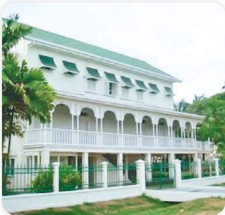
FIGURE 3: TYPICAL URBAN GREAT HOUSE, WITH GROUND FLOOR ENCLOS ED AND SHOWING THE COVERED EXTERIOR GALLERY/ CORRIDOR WITH SUPPORTING COLUMNS (LOGGIA), ORNAMENTAL SPANDRELS AND PIERCED, CARVED BRACKETS
