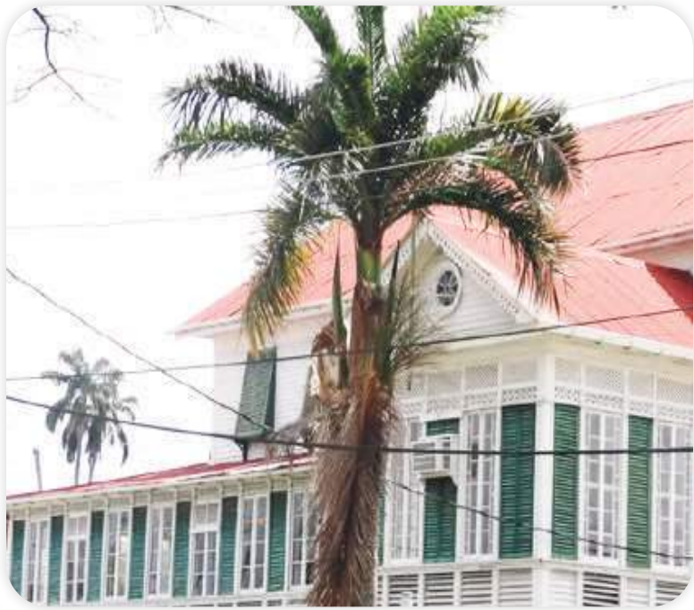
FIGURE 20: ALTERNATING JALOUSIE SHUTTERS AND 8 AND 12-PANED SASH WINDOWS, HISTORIC GEORGETOWN GREAT HOUSE
