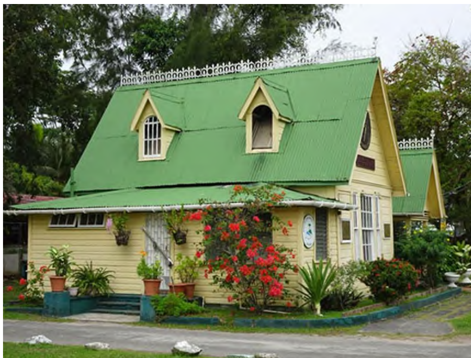
FIGURE 43: IRON CRESTING AND DORMERS ON THE STEEPLY PITCHED ROOF OF JENMANS HOUSE IN GEORGETOWN, 2020
