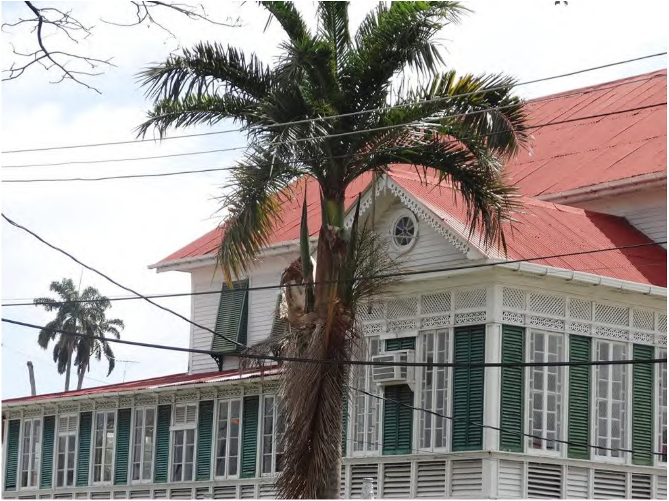
FIGURE 20: ALTERNATING JALOUSIE SHUTTERS AND 8 AND 12-PANED SASH WINDOWS, HISTORIC GEORGETOWN GREAT HOUSE
