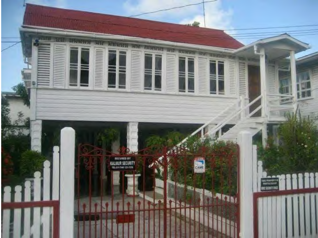
FIGURE 10: WOODEN COTTAGE ON MOULDED CONCRETE BLOCKS, MID- 20TH CENTURY, GEORGETOWN
