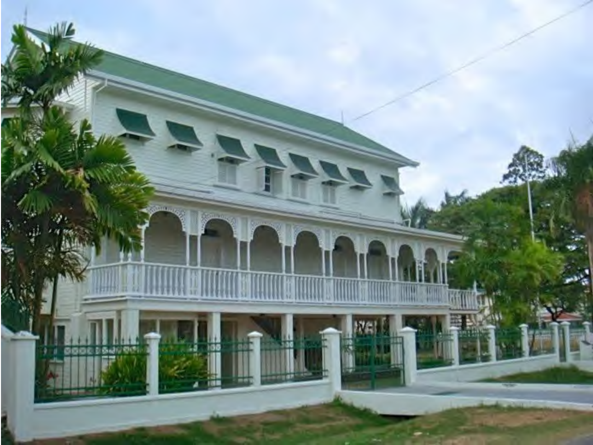
FIGURE 3: TYPICAL URBAN GREAT HOUSE, WITH GROUND FLOOR ENCLOSED AND SHOWING THE COVERED EXTERIOR GALLERY/CORRIDOR WITH SUPPORTING COLUMNS (LOGGIA), ORNAMENTAL SPANDRELS AND PIERCED, CARVED BRACKETS
