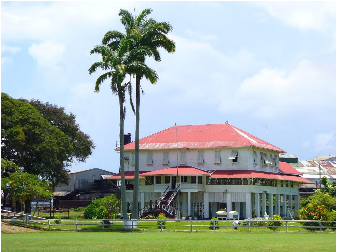
FIGURE 5: TYPICAL RURAL PLANTATION (ESTATE) GREAT HOUSE IN BERBICE, WITH HIPPED ROOF AND ON BRICK PILLARS, BUILT EARLY 20TH CENTURY
